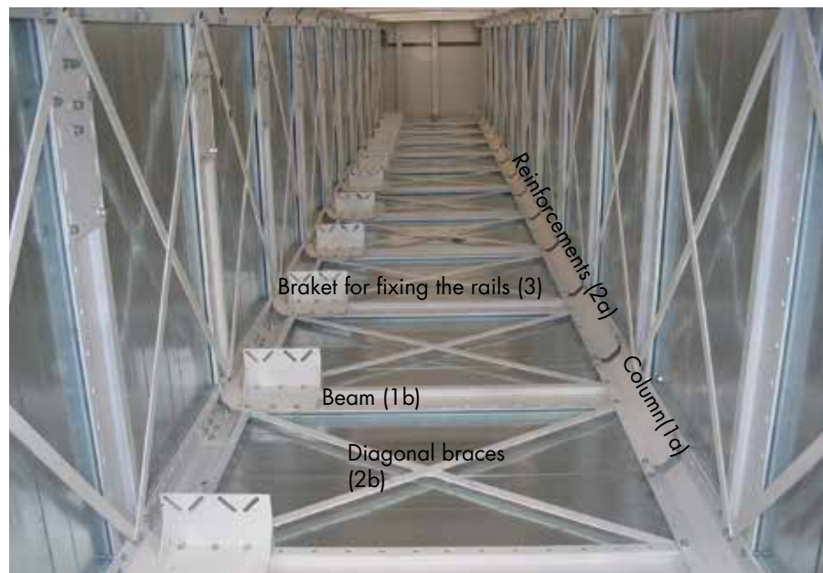
Ill. 2: Components of the DICTATOR lift shaft system
