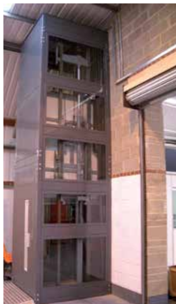
Ill. 4c: Lift shaft with window panes
